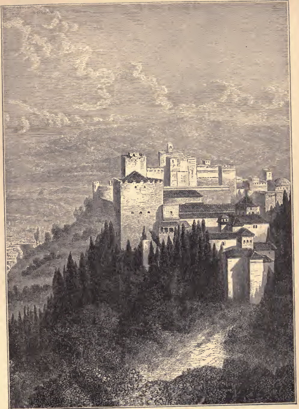
GENERAL VIEW OF THE ALHAMBRA.
